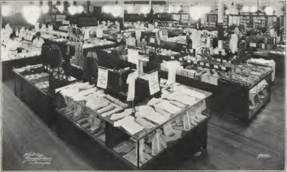
Interior, Grant Store at Tampa, Fla.
